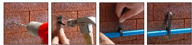
Fixing of Wall Plug Ties.
