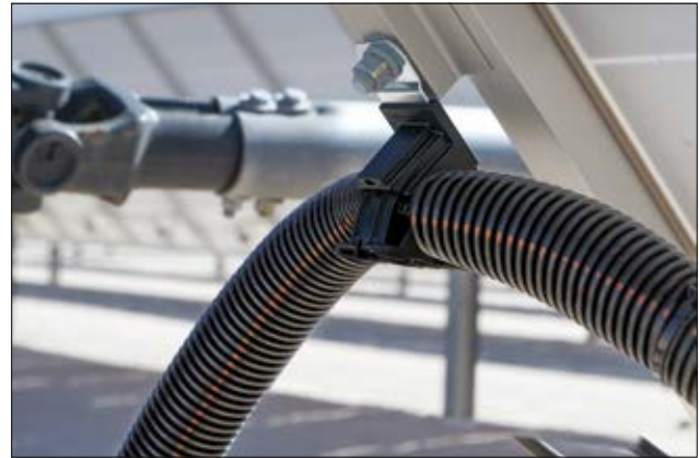
Managing wire in transition on a tracker installation.
